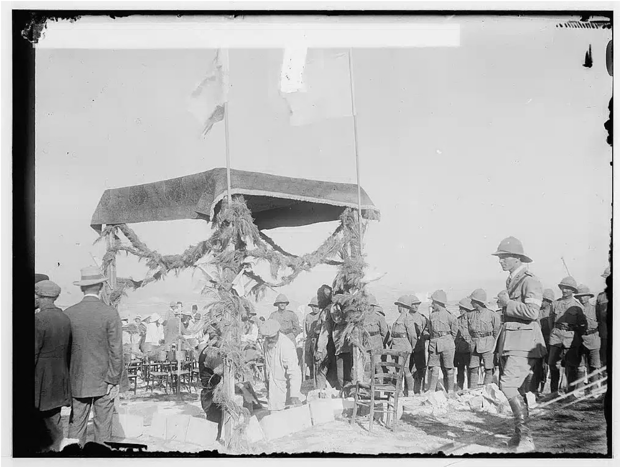
Laying the cornerstone of the Hebrew University during Lord Balfour’s visit in 1918.
